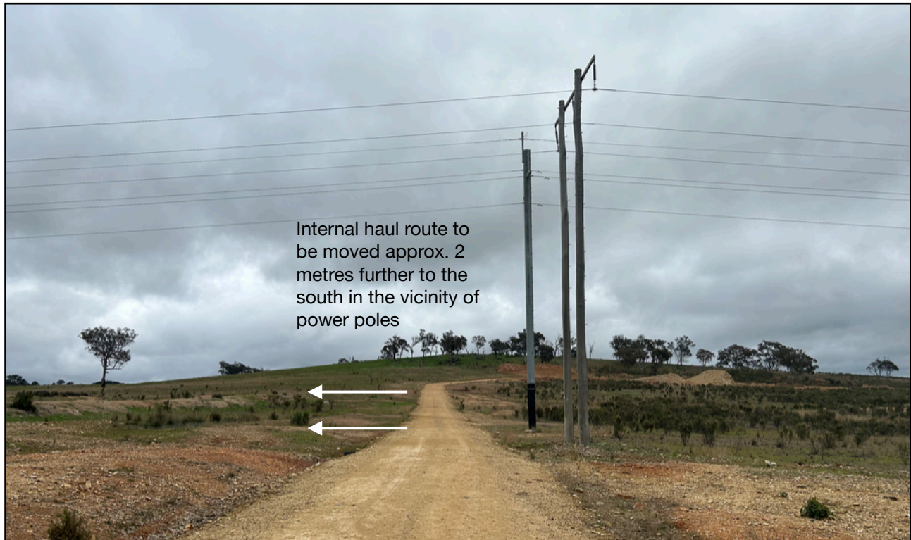
PHOTOGRAPH 3.4: The existing internal quarry haul route will be widened with the route re-aligned 2 metres to the south in the vicinity of the existing power poles that traverse the site. View from near highway entry looking west towards the elevated knoll
